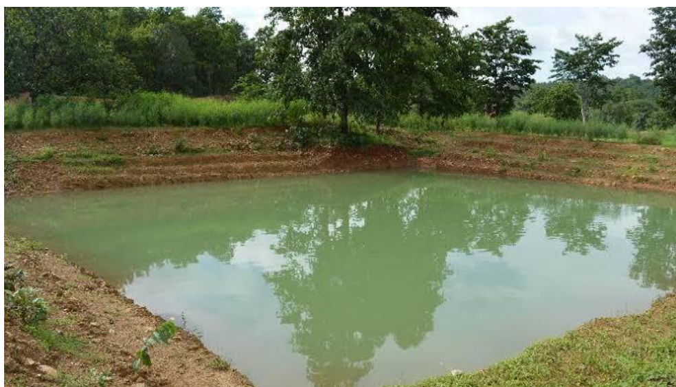
Figure 3. Dobha construction, Photograph by Author
